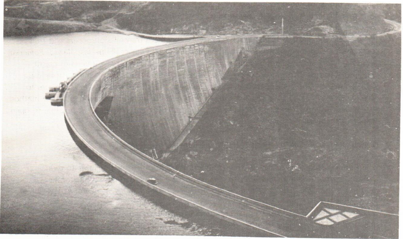
Kariba Dam on the Zambesi River in Central Africa.
