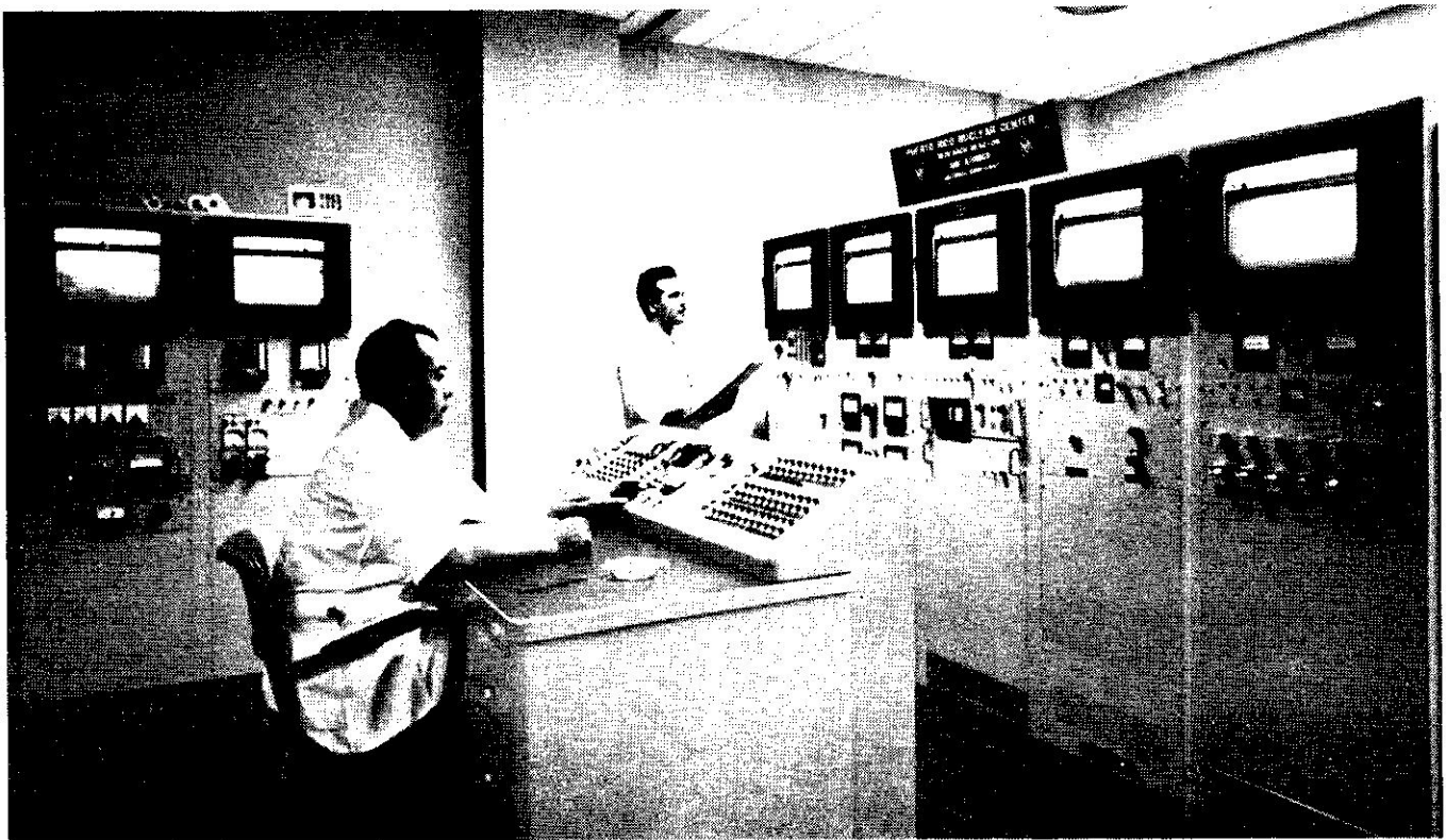
Control room for the PRNC pool type research reactor currently operating at a power level of one megawatt.
