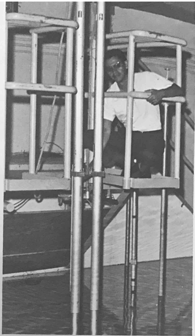
Right: Control rod drives and operating platform for one kilowatt reactor. Below: Reactor control room.
